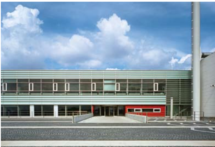
Arkitema K/S: slaughterhouse in Horsens, Denmark
